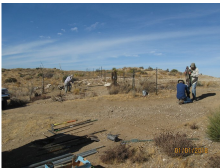
Before - Workgroup Begins Repairs
